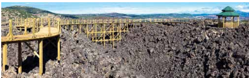
Wooden bridges and park shelters constructed during the project.
