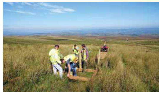
The contractor working on the construction of the boardwalk.
