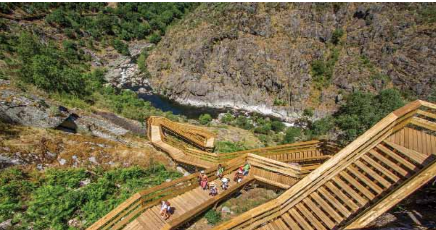
The suspended Paiva River Valley walkway.
