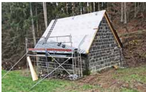
Replacing the roof of the historic pump house.
