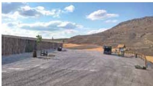
Constructing the interpretive area for the Fuentelsaz Stratotype section.
