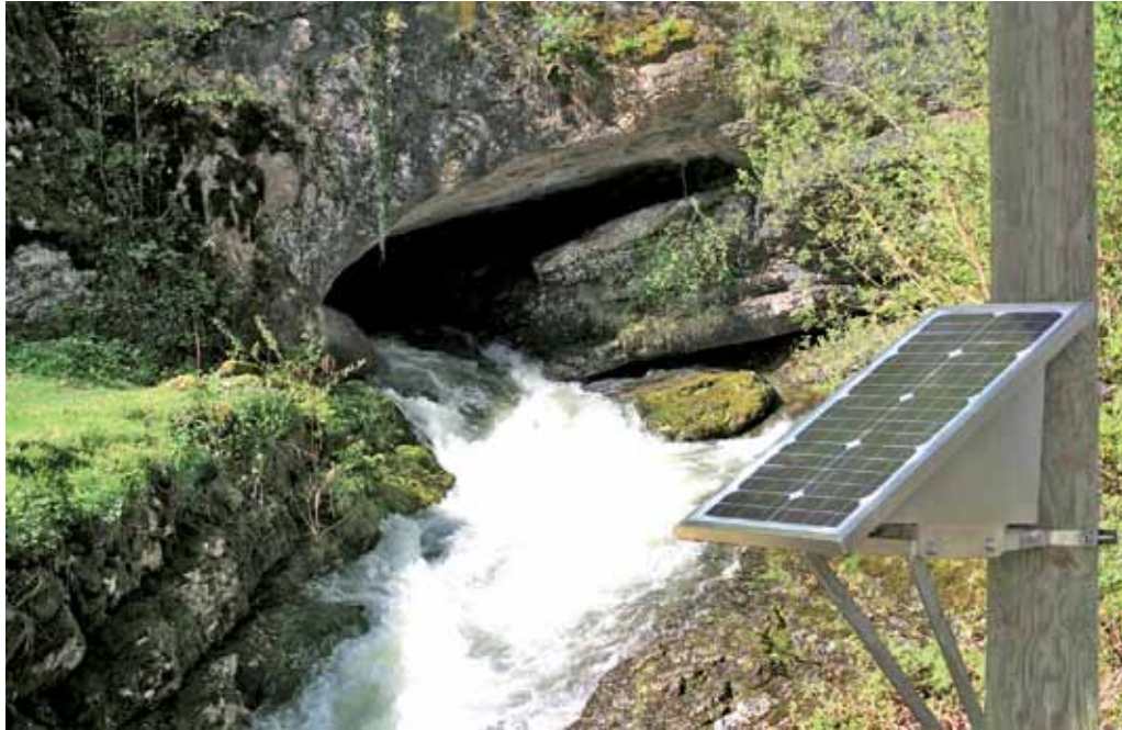
The “Geoborne” on Prerouge Geosite (Solar/ Battery version).
