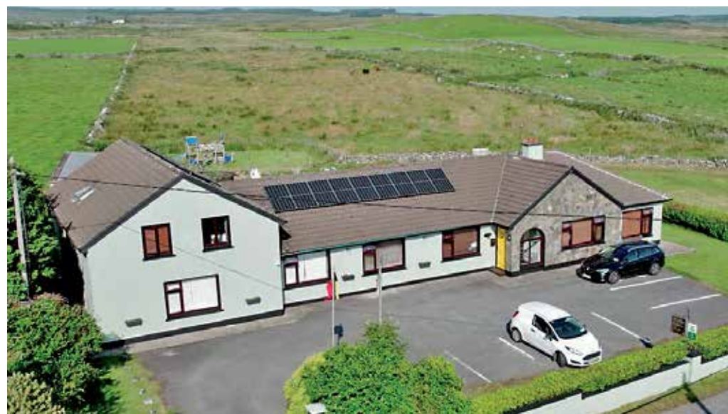
New solar panels installed on the roof of Slieve Elva Bed and Breakfast, one of the 77 members of the Burren Ecotourism Network who have adopted the Geopark Code of Practice.
