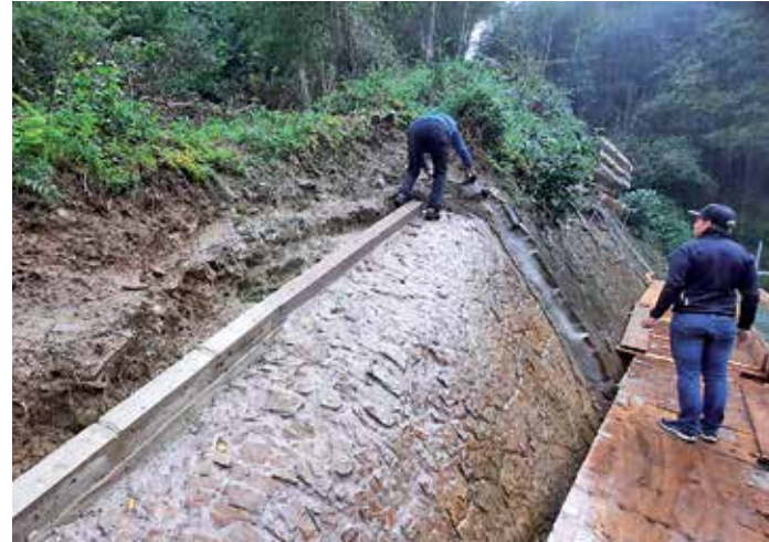
Cementation of the edge of the outcrop.
